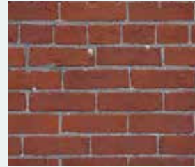
Over-the-Rhine buildings are primarily constructed of handmade, orange-red clay bricks stacked using the common bond pattern, as seen here at 1219 Sycamore Street.
