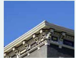
Decorative metal brackets and wood trim form the cornice at 116 West 14th Street.
